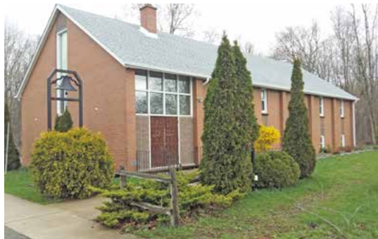
Below: Future roofing: With a new roof All Saints Welland can continue providing their ministry and service in the Dain City area.
