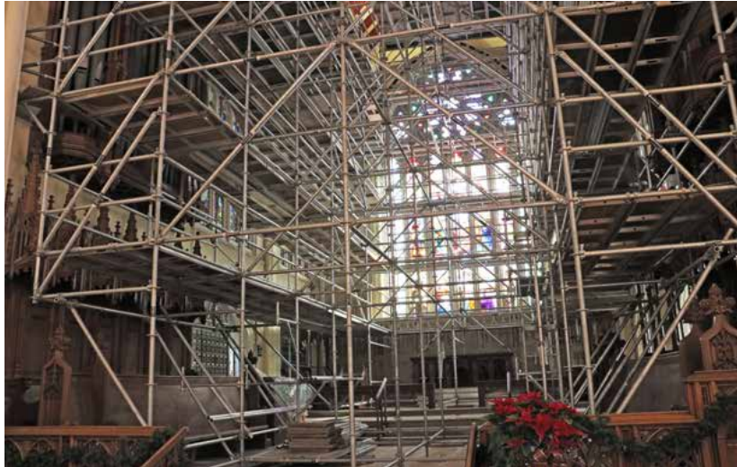
The mammoth scaffolding which enclosed the whole chancel of the Cathedral to allow lighting and safety system upgrades and repair work on the ceiling.
