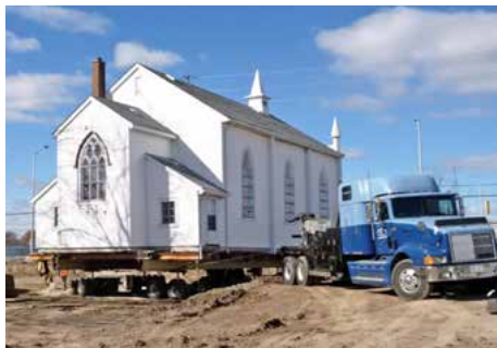
3. Church building is pulled into place.
