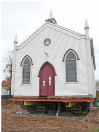
1. St. Luke's is first raised from its foundation, ready to move eastward.
