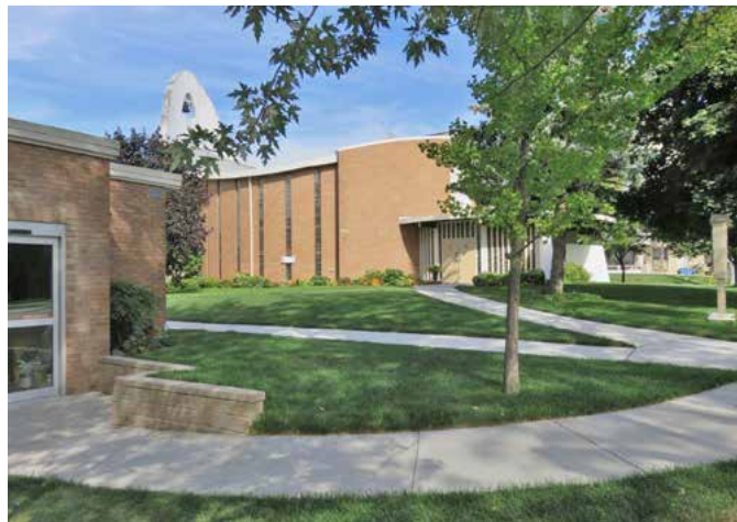
▲ The parish hall and church entrances of St. Michael's Hamilton are now fully accessible after many years of planning and finding funds to complete the job.
