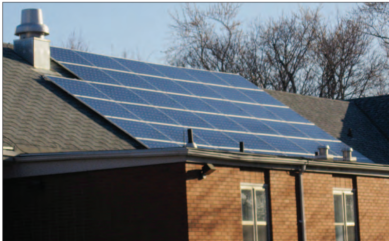
Solar roof completed at Holy Trinity Church, Fonthill
