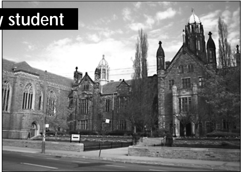
Main entrance to Trinity College (right) with the Chapel (left).
